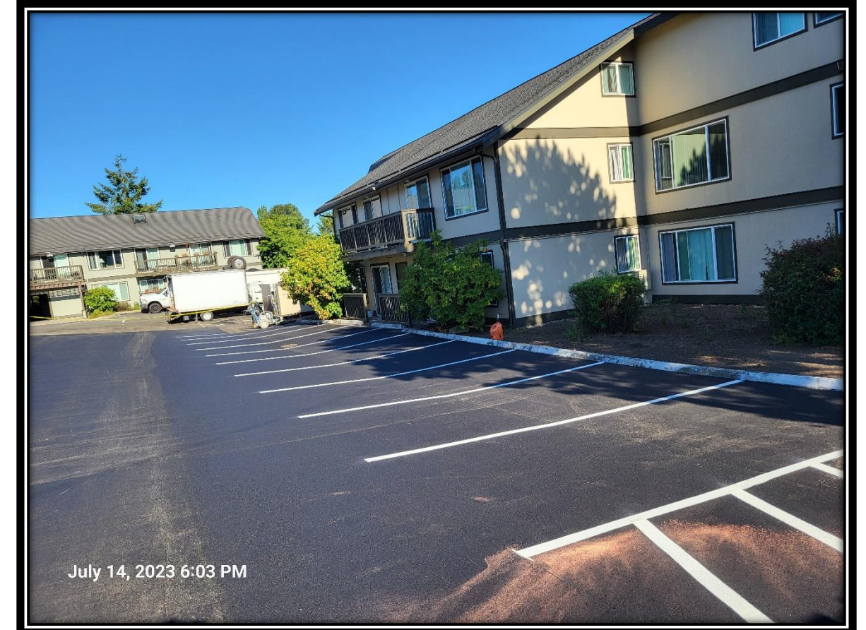
Carriage House Asphalt $39,651
