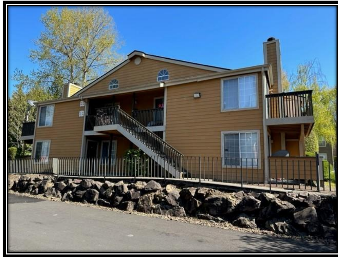
Riverstone Apartments Stairs & Railings $100,000
