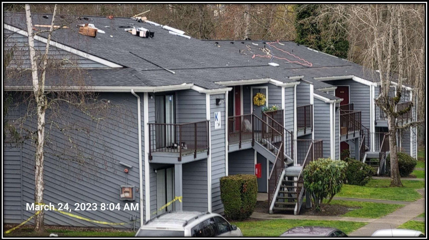
Salish Place Roof $122,250
